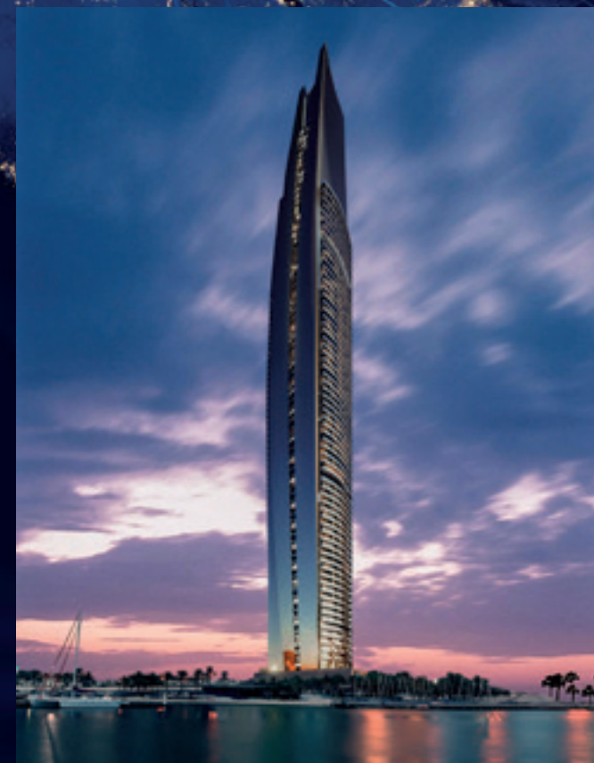
"Damac Height - Fendi Apt" Dubai - (under construction)
